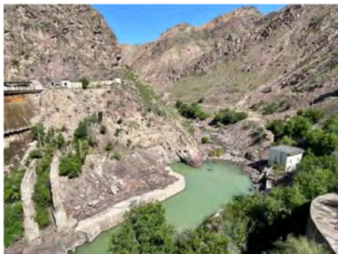
Fig. 3 Scour pit at the downstream
