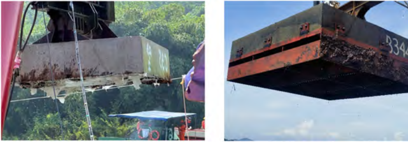
Fig. 1 Concrete anchors vs shear key anchors
