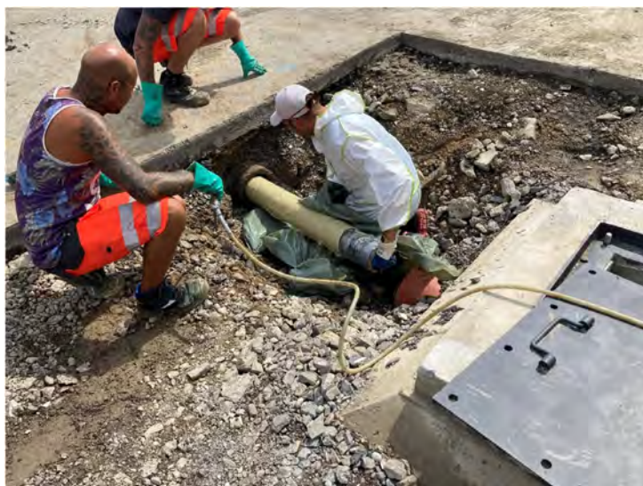
Fig. 9 Installation of shortliner Installation de chemisage partiel
