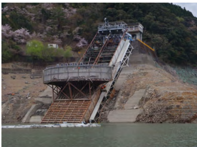
Fig. 4 Selective water intake facility Installation de prise d'eau selective
