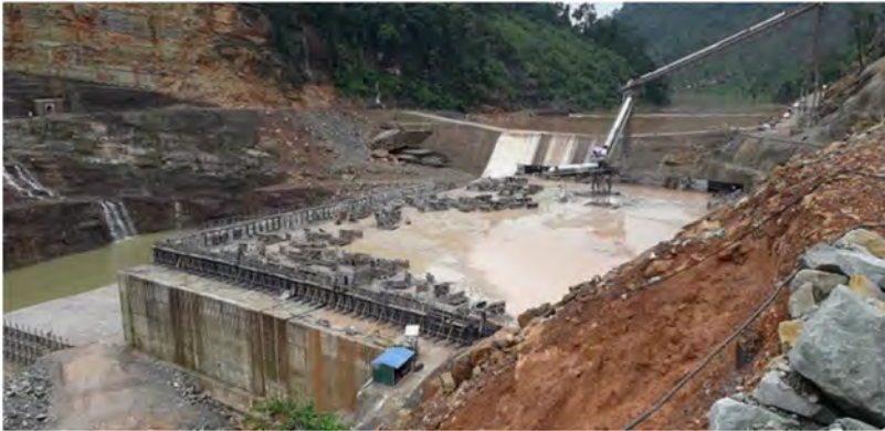
Fig. 7. Overtopping of Upstream RCC Cofferdam and Main Dam on 16 August 2019
