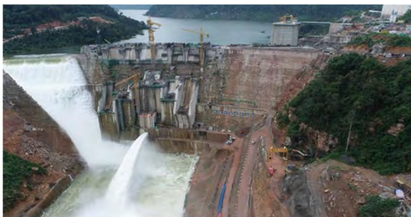
Fig. 9 Overtopping of RCC dam on 11 August 2021 ( Q_{in} = 3,878 \text{ m}^3/\text{s} , Annual Flood)
