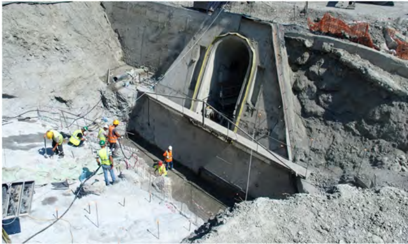
Fig. 5 Construction of the Dam Gallery
