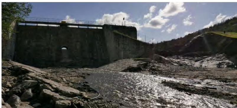
Fig. 4 View of the cross-section of the dam breach in Stronie Śląskie.
