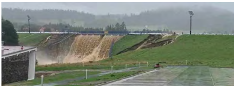
Fig. 3 The dam in Stronie Śląskie after the failure, viewed from the airside.
