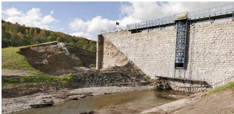
Fig. 2 The initial phase of the dam failure in Stronie Śląskie (source: user @aborowicz, platform X)
