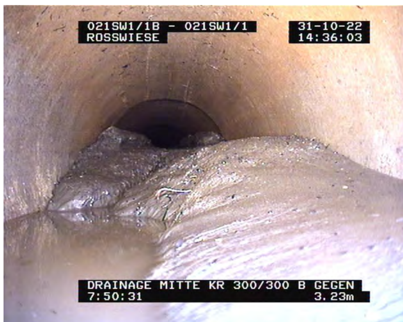
Fig. 6 Drainage pipe, filled with sediments tuyau de drainage, rempli de sédiments
