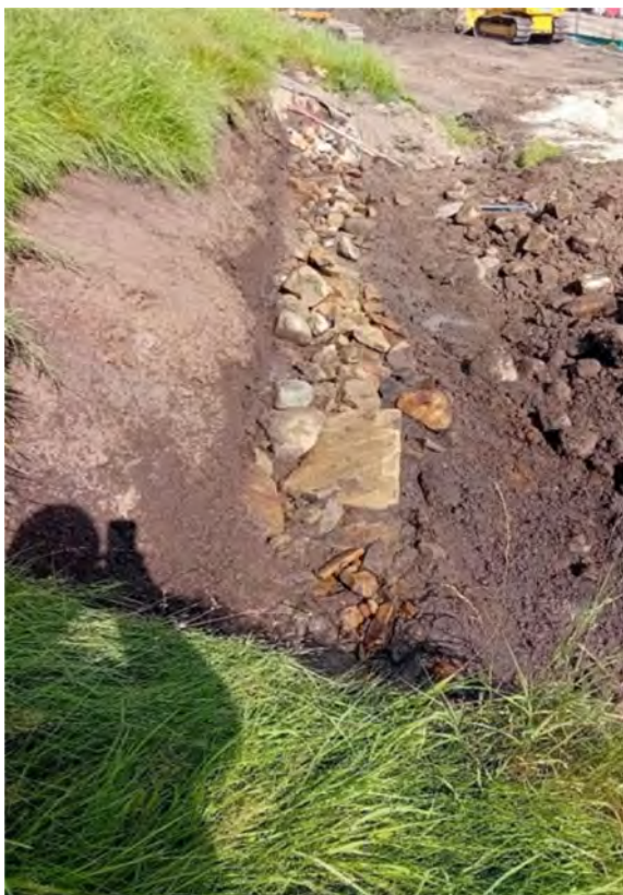
Fig. 2 Example of wall drain in downstream shoulder at Barrowford reservoir
