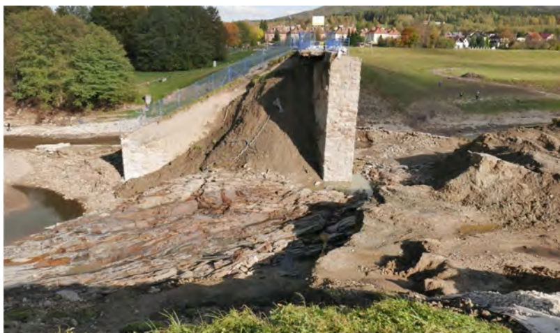
Fig. 5 The dam in Stronie Śląskie after the failure, viewed from the waterside.
