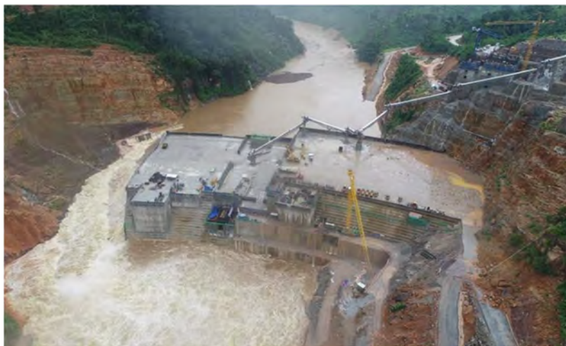
Fig. 8 Overtopping of RCC Dam on 02 August 2020 ( Q_{in} = 2,110 \text{ m}^3/\text{s} )
