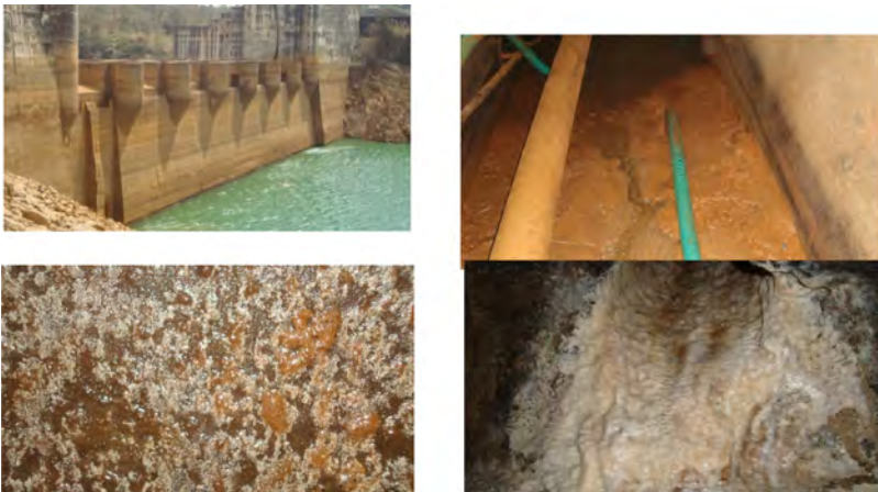
Fig. 3 Effect of acidic reservoir water and condition of drainage galleries
