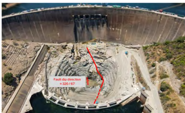
Fig. 6 Trace of the main fault across the excavation
