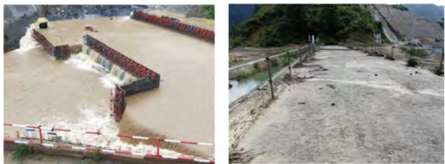
Fig. 3 Xijiang dam under overflow and after overflow during construction
