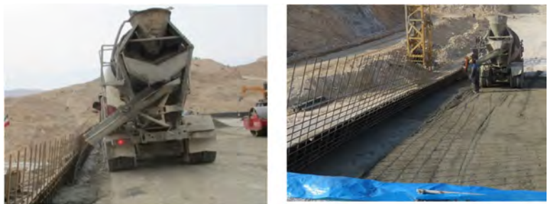
Fig. 3 Reinforced conventional concrete against RCC system in upstream face of Baghan dam
