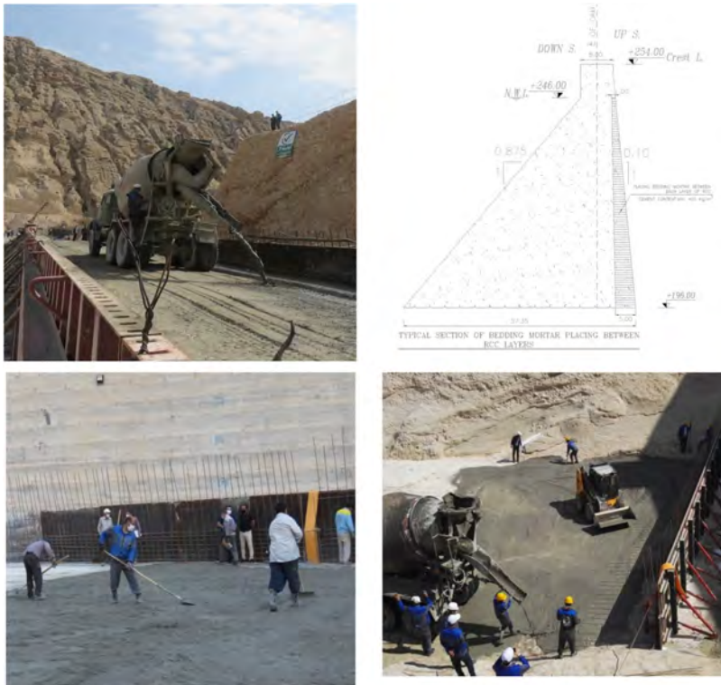
Fig. 4 Interlayer bedding mortar placement during construction of Baghan RCC dam
