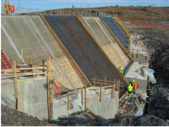
Fig. 6 Reinforcement in place on two upstream slabs.
