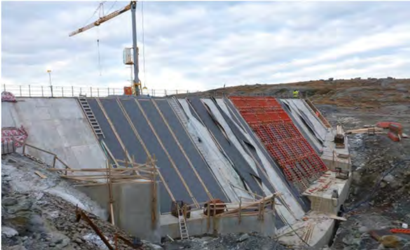
Fig. 7 New slab on the upstream side. Insulation cover of the concrete during hydration was necessary due to the cold climate in the late autumn.
