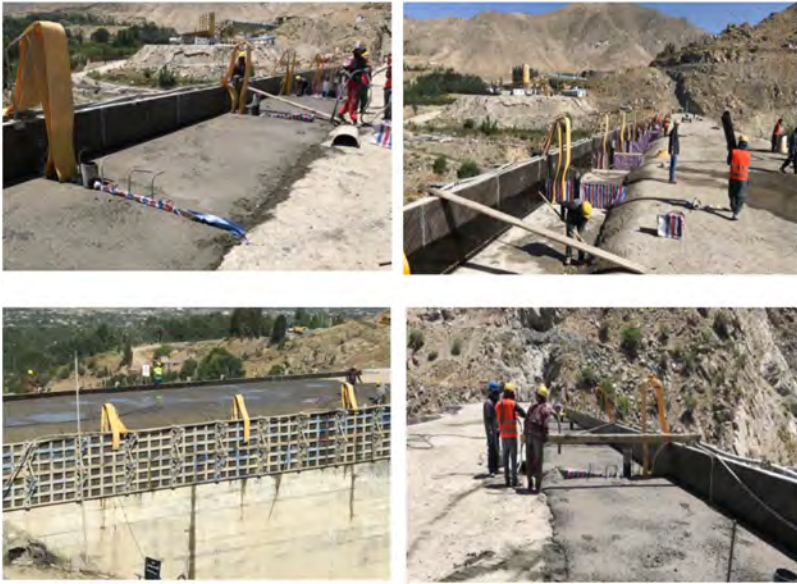
Fig. 1 Construction of upstream face of SHAH-WA-ARUS dam
