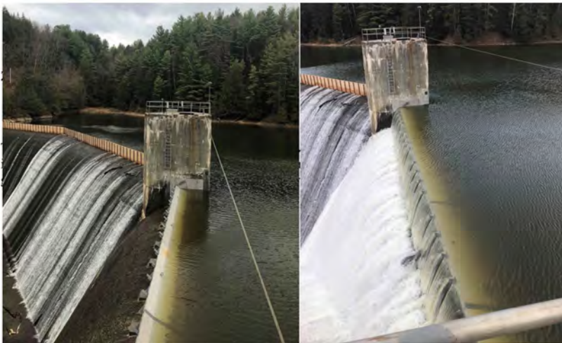
Fig. 7 Installation of Modified Crest Gate
