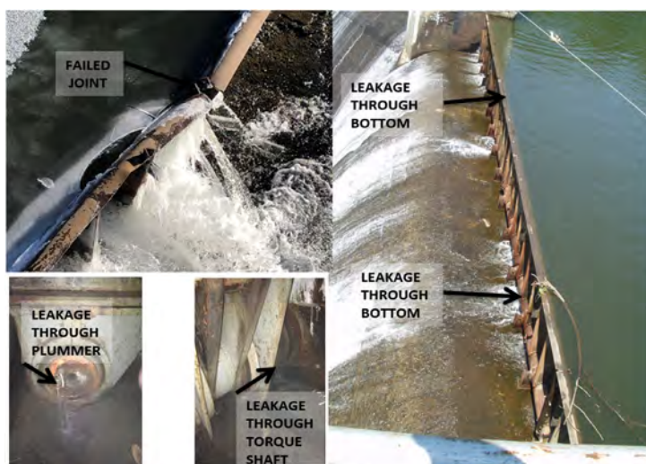
Fig. 4 Failed Joint & Leakage through Existing Crest Gate
