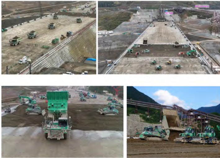
Upper: Overview of CSG concrete construction, Lower left: Unloading and spreading by AAC Dumps truck and AAC Bulldozers, Lower right: Compaction by AAC rollers
